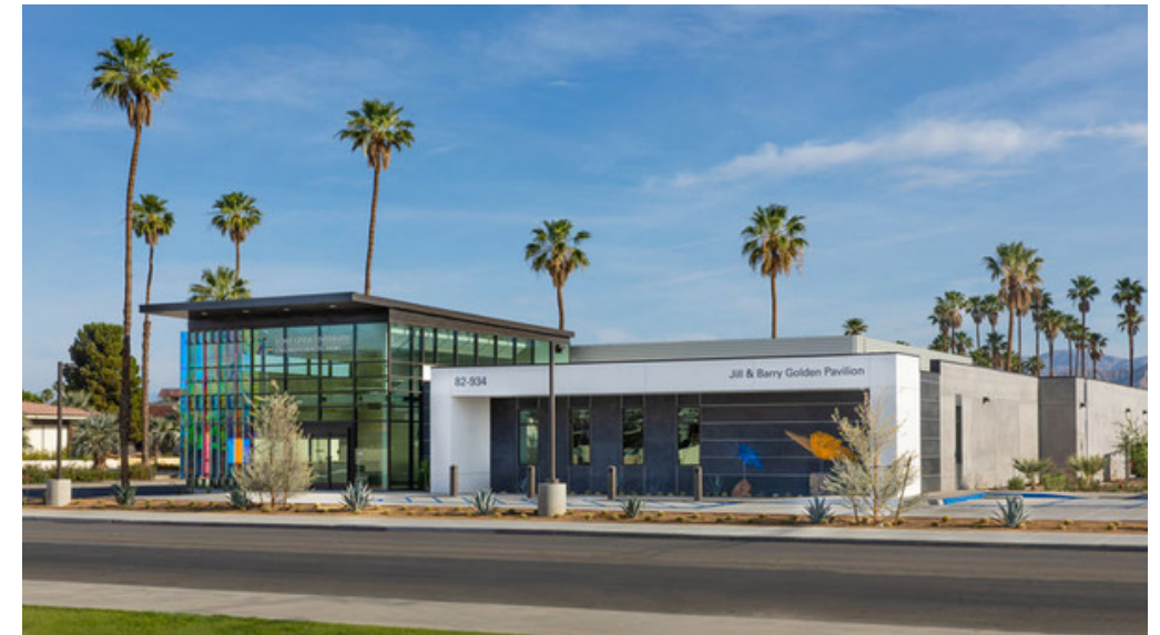
Loma Linda University Children's Hospital Indio, CA Location.
